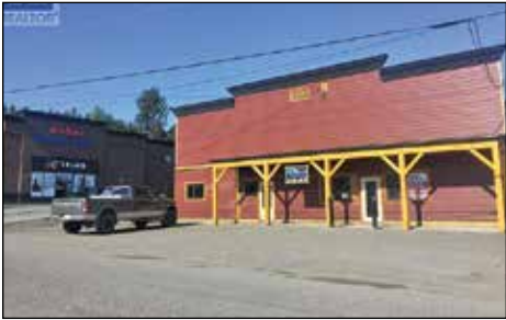
MLS C8034548 $359,000 Commercial building approx. 3,600 sq. ft. plus approx. 600 sq.ft. lean-to at the back. Unfinished attic which has the potential for further development. Located in a great spot with excellent highway exposure. Zoned C-3 which includes a variety of different uses - restaurant, office, hotel, motel, retail sales, etc., etc. FR L0042 100 Mile House
